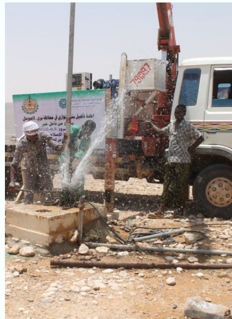
Rehabilitation of borehole
